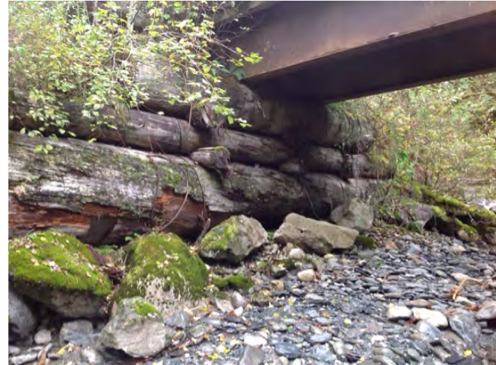
Right Bank Abutment when facing downstream
