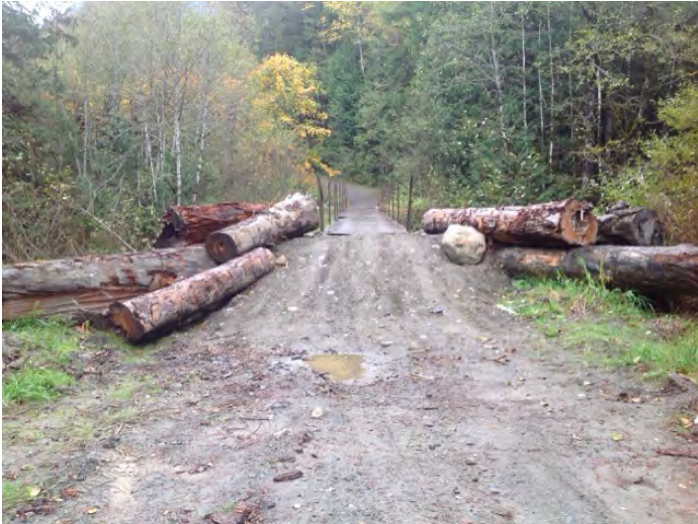
Approach from Left Bank when facing downstream
