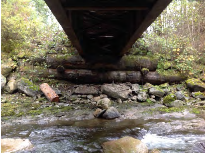
Left Bank Abutment when facing downstream
